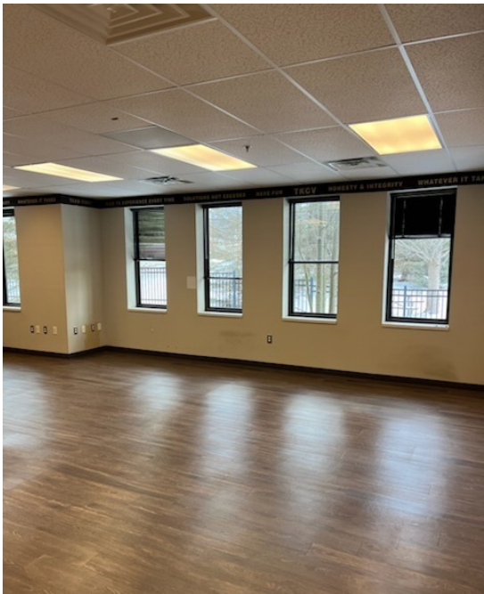
Main Level - Photo 3
